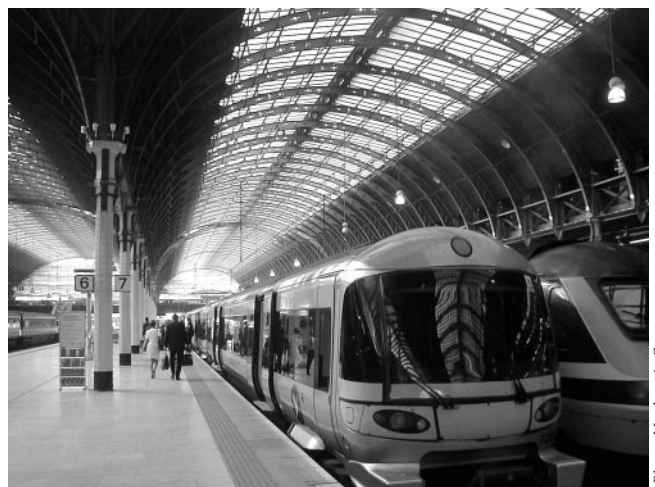
Figure 5-4. The Heathrow Express at Paddington Station.
