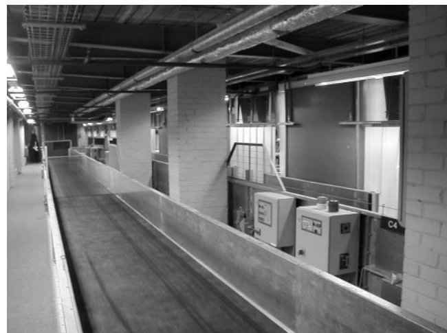
Figure 5-31. The bag is sent on a conveyor belt under the platform to the head of the train.
