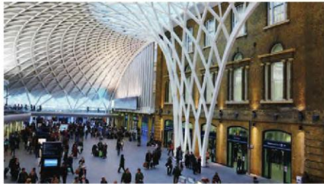
b After renovation
