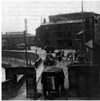
a Before renovation
