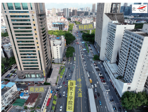
图4 中山大道“天府路—科韵路路段”改造前情况 Fig.4 Pre-renovation conditions of Zhongshan Avenue (Tianfu road-Keyun road section)
