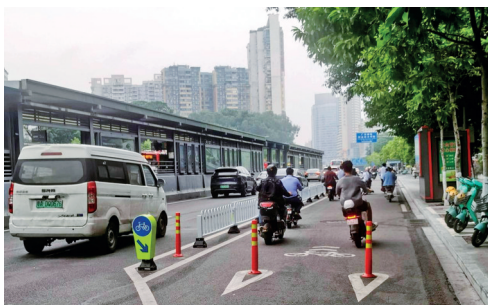
图5 类型I设计模式：机动车道缩减与非机动车道拓宽 Fig.5 Design type I: reduction of motorized vehicle lanes and expansion of non-motorized lanes
